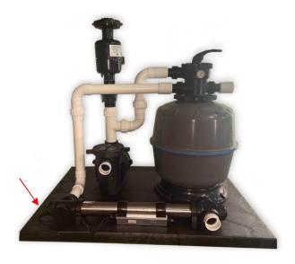
Step 1: Start by laying the Pad on level ground where you want to locate the equipment.
