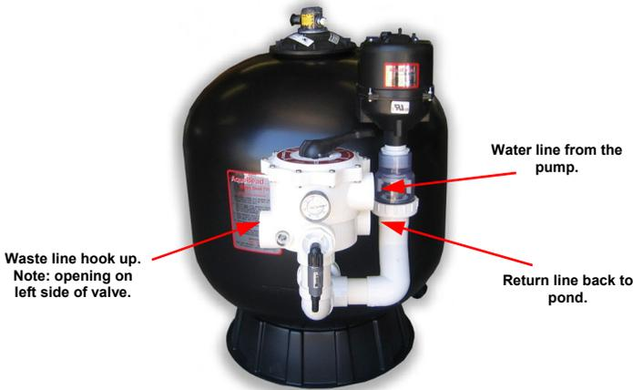
Make plumbing hook ups as shown in the picture. Use 2" male threaded adapters to thread into the open ports of the Multiport valve and then use unions to secure plumbing to valve.
