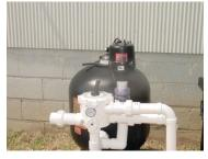
Step 9:Place Bead Agitator onto AquaBead filter.
