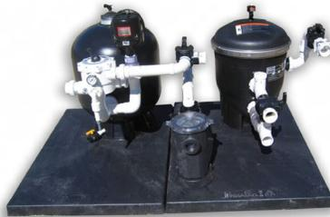
Step 9: Attach "Vortek SS Bypass" As shown.
