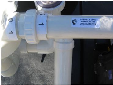
Step 7: It's now time to assemble the pipework. This part is done simply by hand tightening (ONLY) the connections of "LIKE NUMBER TO LIKE NUMBER" such as 1 to 1 and 2 to 2 etc.
